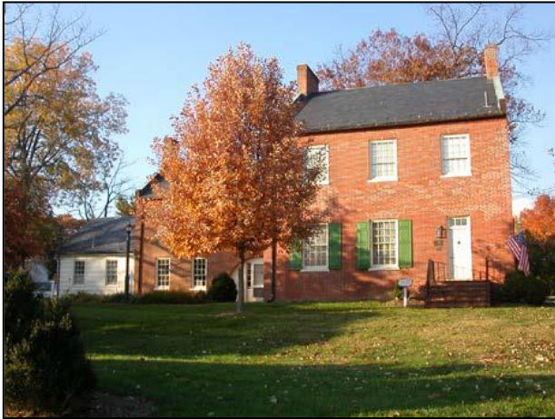
Beall-Dawson House at 103 W. Montgomery Avenue
