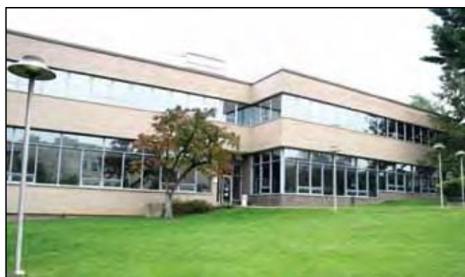
Former Rockville Library, 99 Maryland Avenue, demolished in 2009
