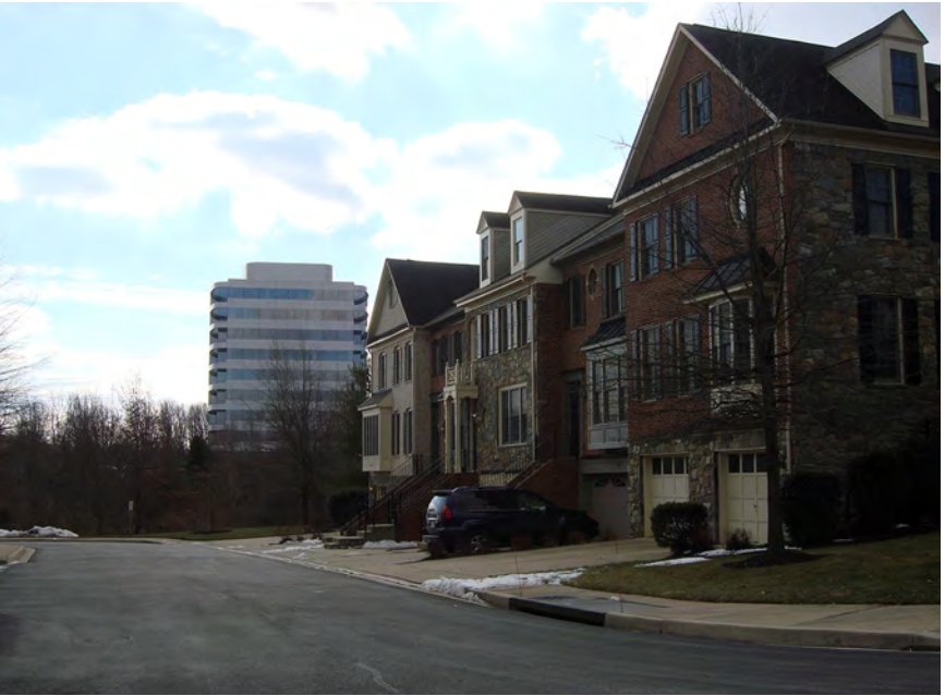
The Tower Oaks development is a hybrid of suburban and urban forms, including multistory office buildings surrounded by parking and rowhouse style townhouses with stoops and front facing garage doors and parking aprons.
