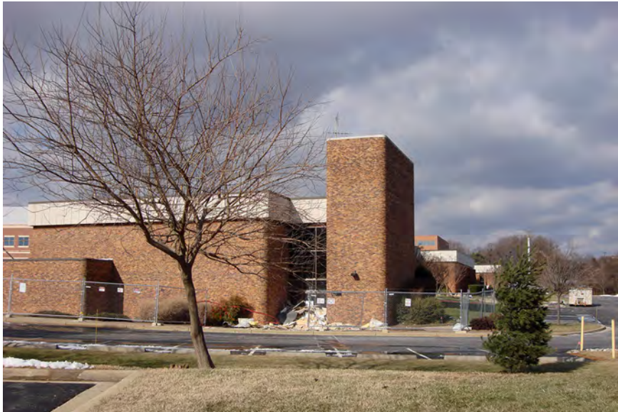
Laboratory building, at the south end of Research Boulevard, built in the mid 1960s under demolition in 2015. The current proposal is to convert the property to a retail use with fitness center and shops.
