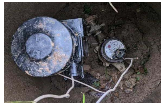
Sanitary sewer main with root in joint defect that requires rehabilitation (top); water meter and appurtenances (bottom)
